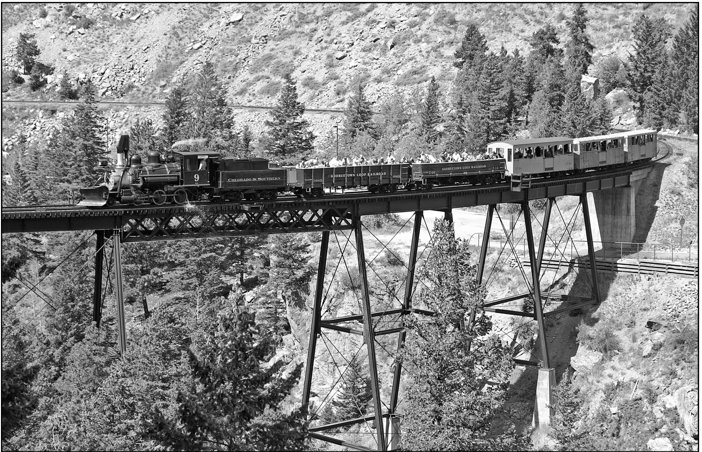
Recently restored Colorado & Southern locomotive No. 9 climbs across the Devils Gate High Bridge on the Georgetown Loop Railroad on September 1, 2006. – Three photos © 2006 Dave Schaaf
