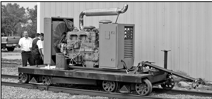
Power for D&IM No. 25 is provided by this diesel generator set. – Photo © 2006 Dave Schaaf
